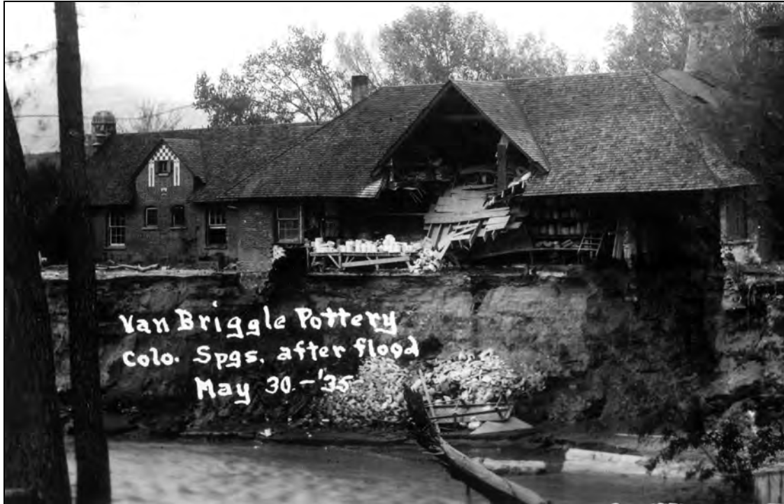
Figure H14. The 1935 Memorial Day flood of Monument Creek severely damaged the pottery's molding/casting wing and left water, sand, and mud throughout the rest of the plant. SOURCE: Colorado Springs Museum, Starsmore Center for Local History, Van Briggle photographic collection, accession number S 2000.0143.0001.
