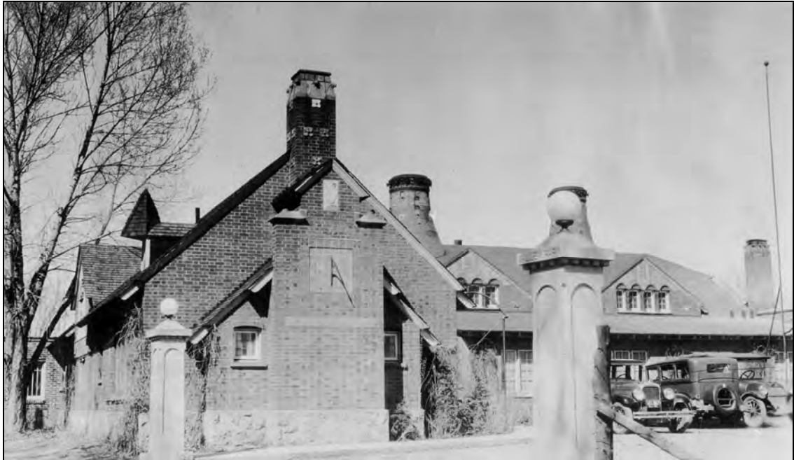
Figure H13. A variety of tile installations with the theme of time appear in this 1920s view of the west wing. SOURCE: Colorado College, Facility Services Department, Miles Schmidt collection.
